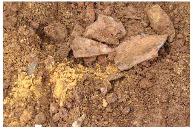
Figure 1 Asbestos cement fragments in soil.
